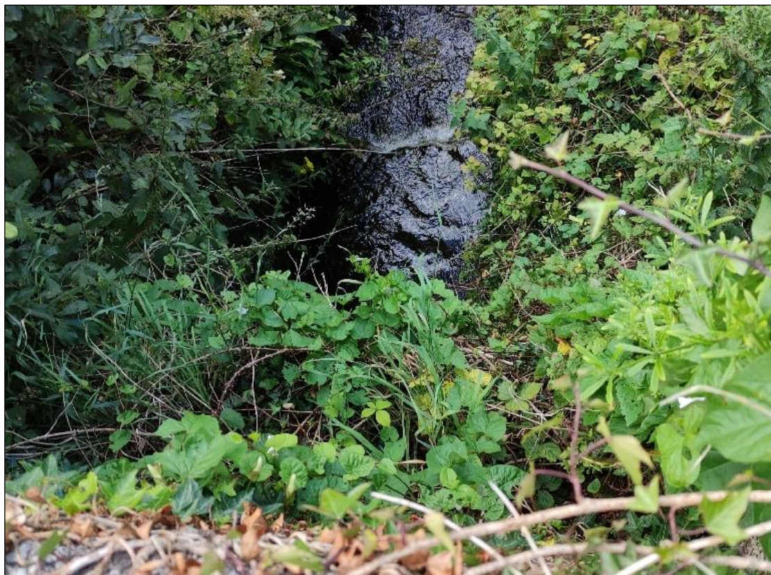
Plate 6-29 Unnamed stream beneath the road at water crossing 5
