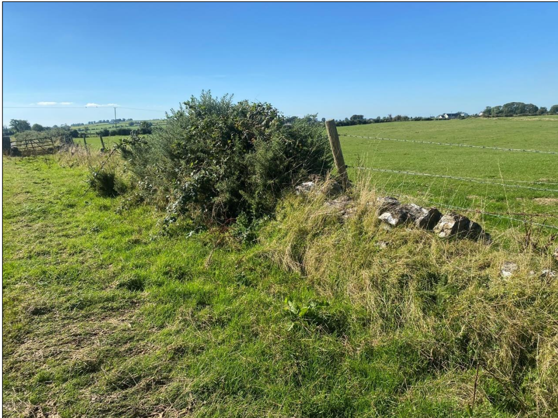
Plate 6-23 Stone wall (BL1) within the Proposed Wind Farm site
