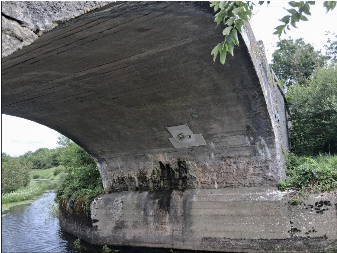
Plate 6-32 Water crossing point 8 along the Proposed Grid Connection
